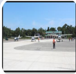
AIRPORT IN SAN JUAN DE NICARAGUA (RIO SAN JUAN)
