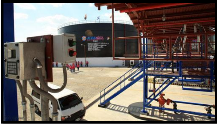
Storage complex in Corinto
